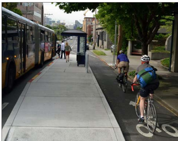
Bus bulb-out with bike lane behind: Seattle, WA
